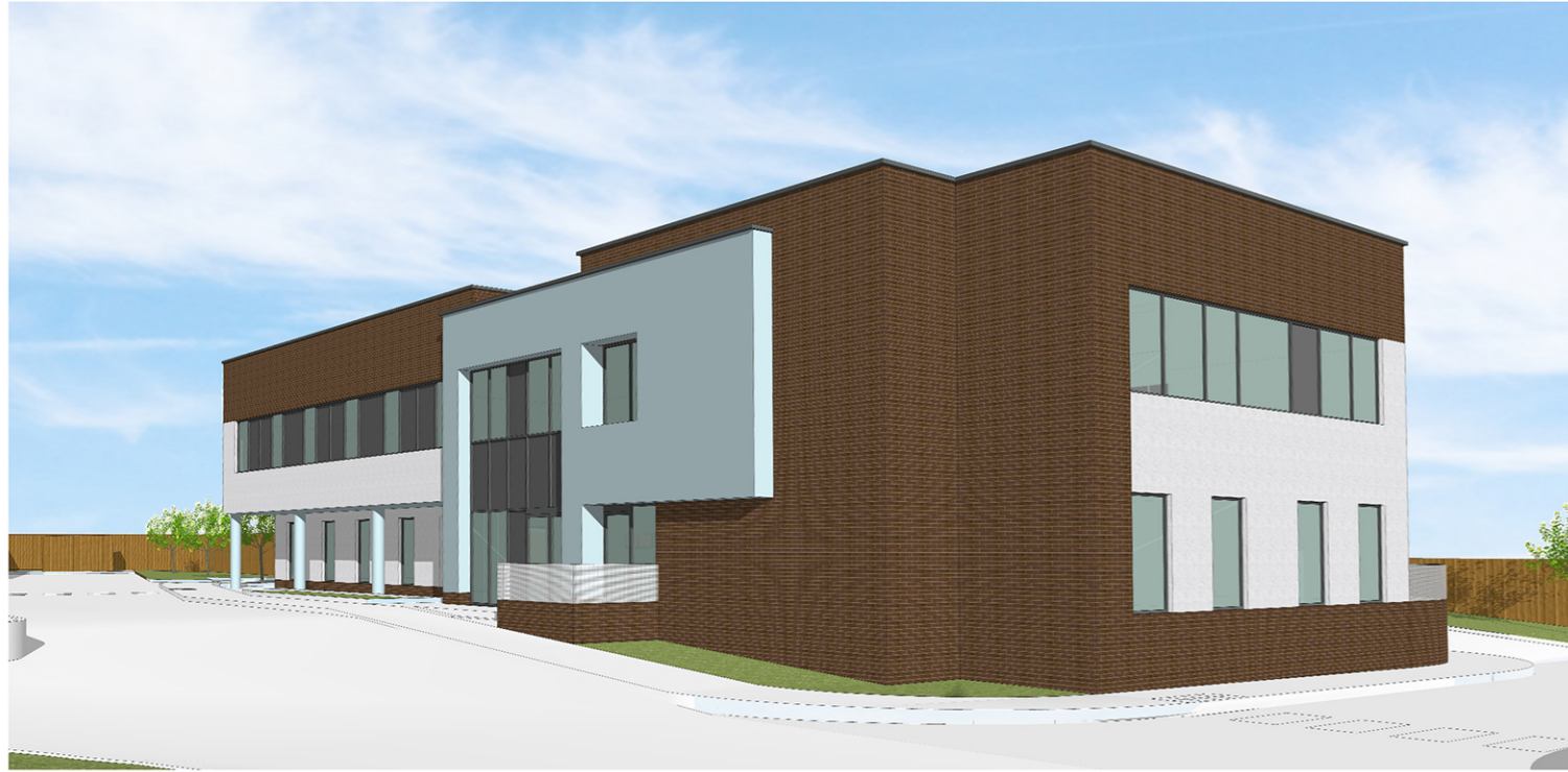
North West View
